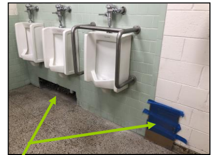
Cut-outs in the cinder block wall to repair the leaks
